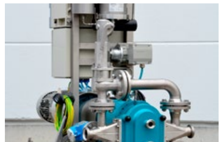
Overpressure protection by bypass with safety valve
