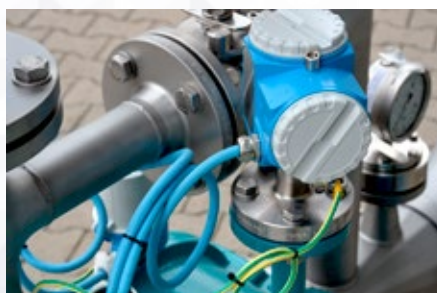
Electronic leak monitor
