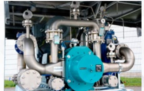
Variocap as mechanical overpressure protection
