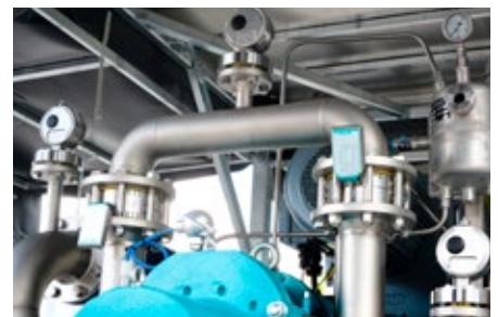
Overpressure protection by bypass with rupture disks
